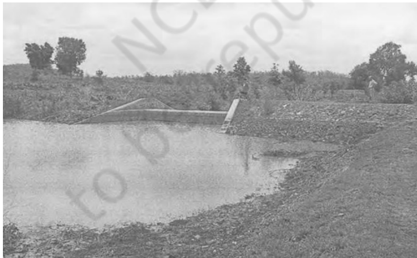
A small dam
